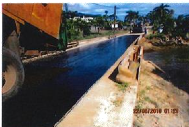
Chip Sealing – Bituminous Surfacing
